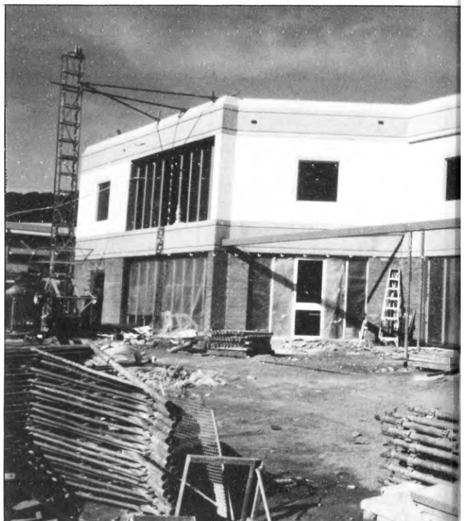
2. Rear view of the building.
