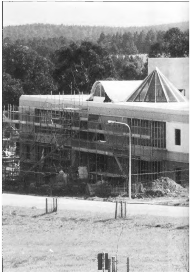
1. View of the front of the building.
