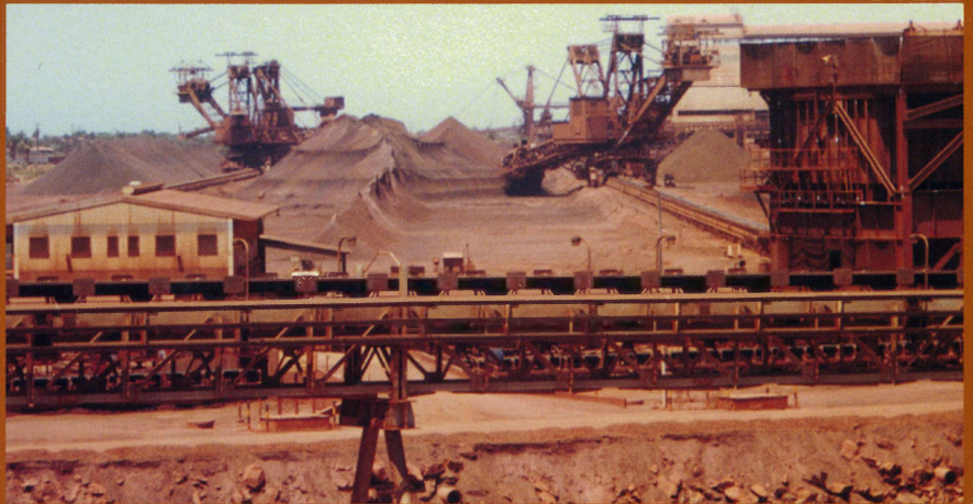
Huge loading yards, such as this iron ore storage, keep the Pilbara ports busy day and night.
