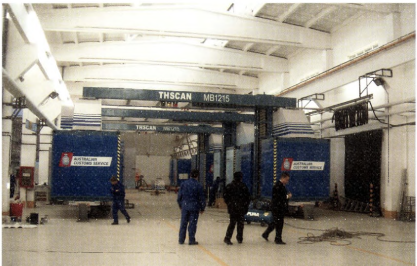
Container x-ray system construction in China.
