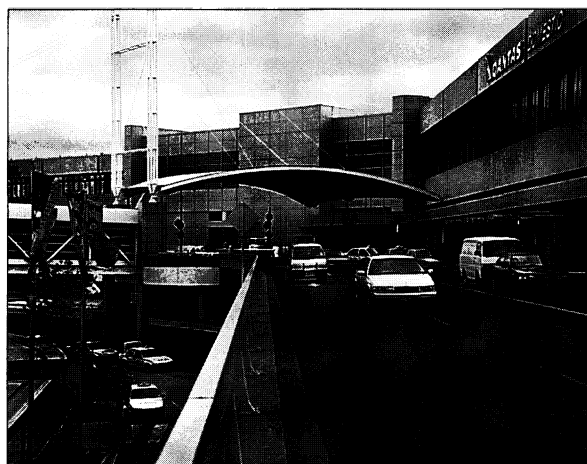
Photography by Arthur Mostead
